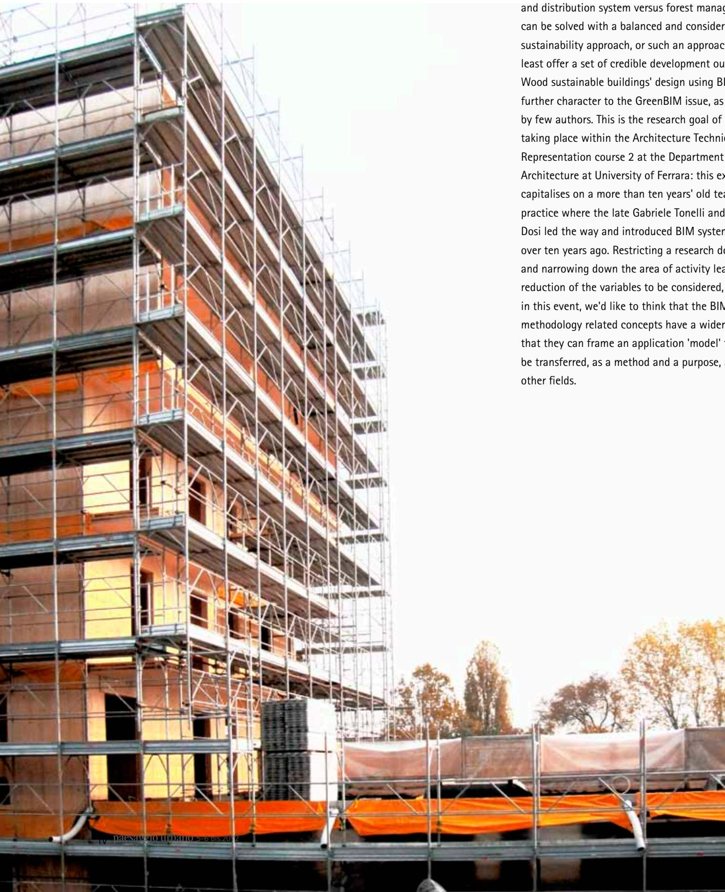
View of the D tower in Via Cenni during the upper floors' completion phase. The structure is made by two 2-storey blocks delimiting a green court, and four 9-storey towers raising from the main buildings.
